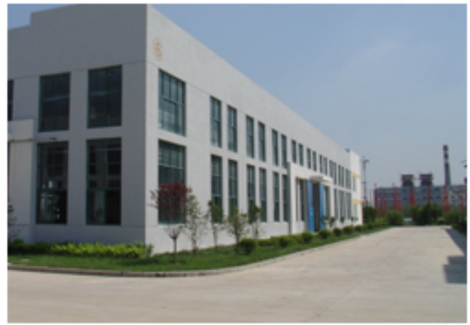
Our Chintec plant is strategically located in a “high technology zone” in Wuxi, China.
